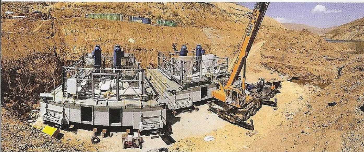
Pontoon assembly adjacent to the tailings dam at Sungun mine.
